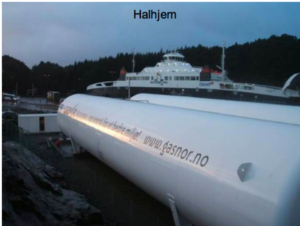
Figure 5-4: LNG semi-permanent refueling station for LNG-fueled ferry (Norway). LNG refueling station for the Fjord1 ferry. The ferry operates on a fixed route to Halhjem, Norway. The refueling facility is a semi-permanent LNG tank structure (Skjervheim, 16).
