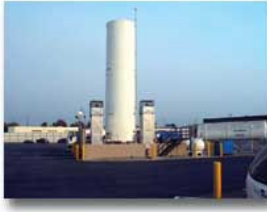
Figure 5-9: LNG onshore vertical storage tank (United States). An onshore LNG vertical storage tank in the United States (California Energy Commission).
