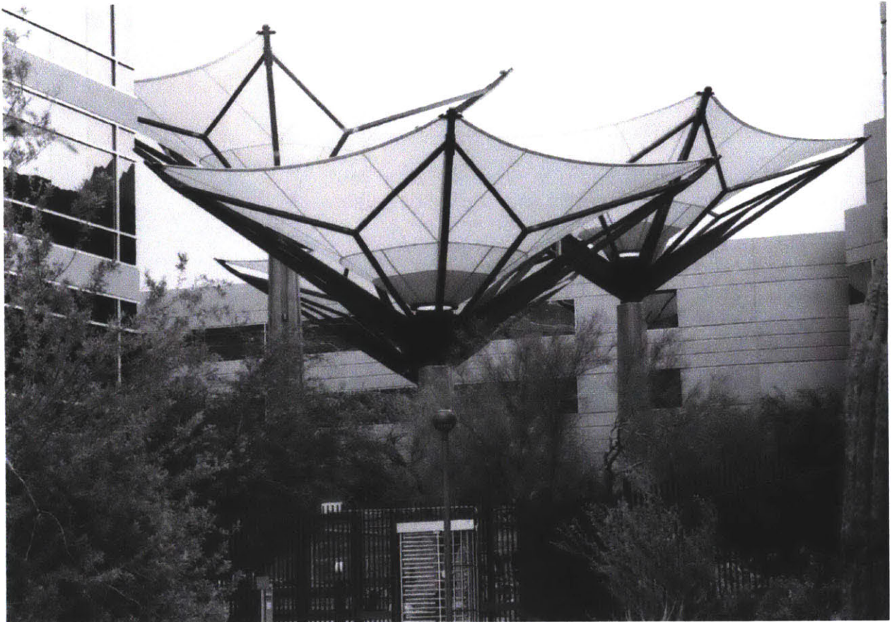
Heather Kinkade-Levario, Raincatching, shade-roviding, upside-down ubrellas in a central courtyard of multiple commercial office buildings , 82, JPEG
