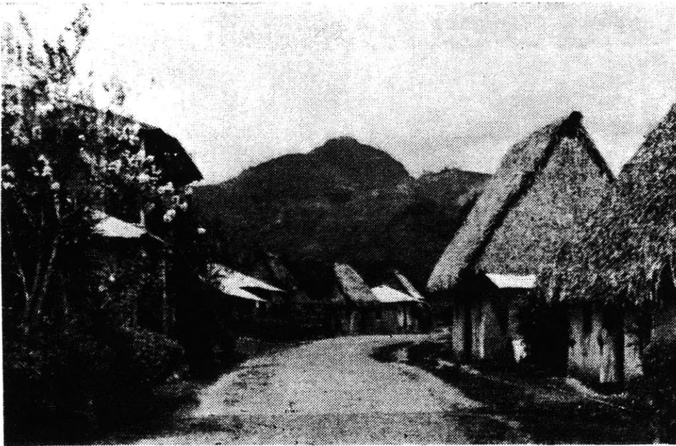
Fig. III.11. Wooden structure (above) of traditional wattle and daub construction (lower) in Panama.
