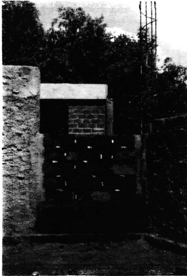
Fig. IV.4. Earth-block wall in Auroville, India, with protruding pieces of stone chips to provide bonding with the cement plaster to be applied.
