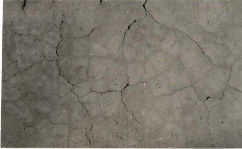
Figure 24. Photograph of surface (Batch #26, 15 cycles, 1.7X) of quenched alumina-titania brick. Macroscopic cracks are to be distinguished from the faint microscopic cracks. Note that while significant macroscopic cracking appear, those cracks do not run across the dimension of the brick.
